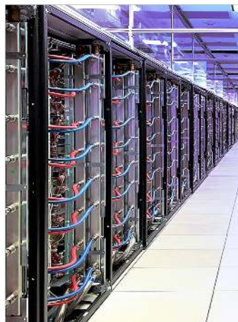
Direct-to-Chip Liquid Cooling
